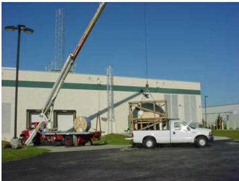
Lifting antennas onto the RDC roof.
